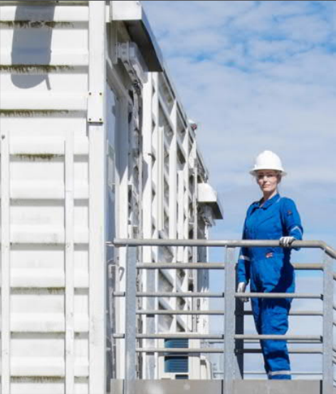
Stationary Energy Storage
